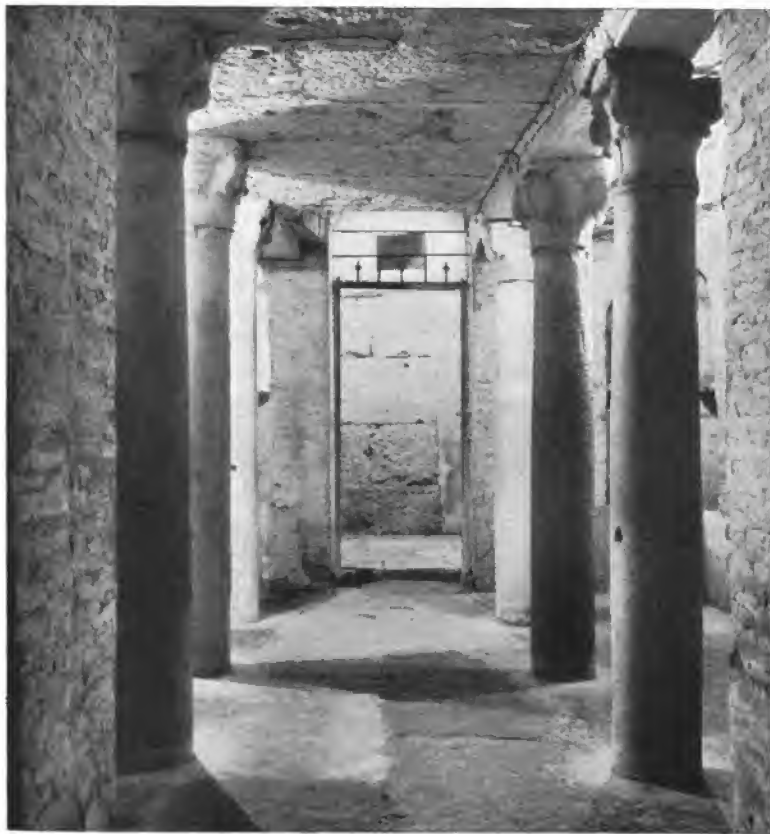
Fig. 234 — S. Maria in Cosmedin. Interior of the crypt, facing west (Photo: E. Nash).
